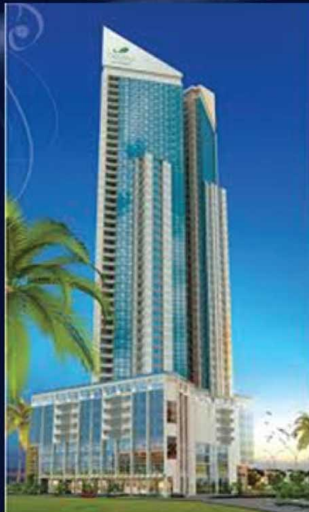
Plumbing & Electrical Contractor for Destiny Mall & Residencies Project (On-going)
