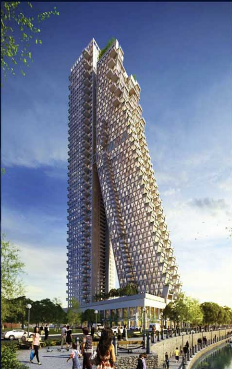
Plumbing Contractor for Altair Residential Development Project (On-going)
