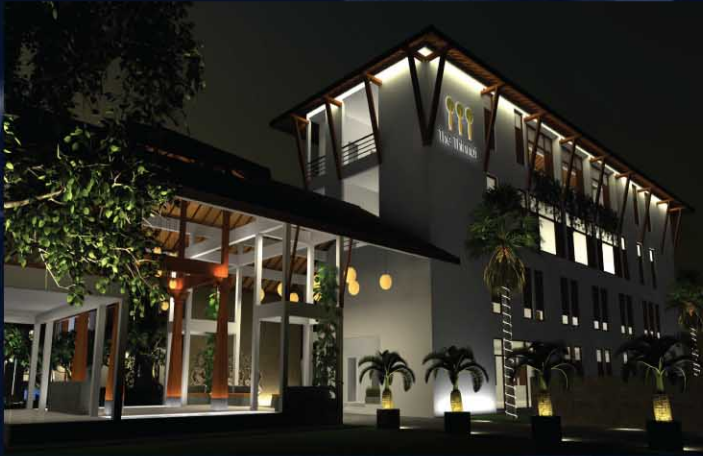
Mechanical, Electrical & Plumbing Contractor for The Thinnai Hotel - Jaffna (Completed)
