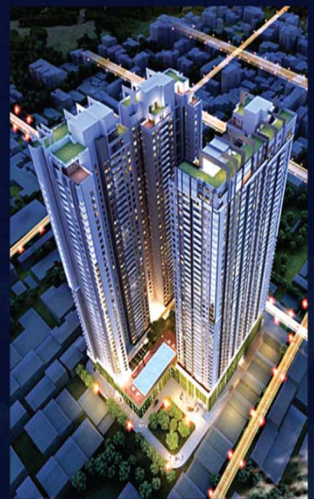
ELV Contractor for Avic Astoria Residential Development Project (On-going)
